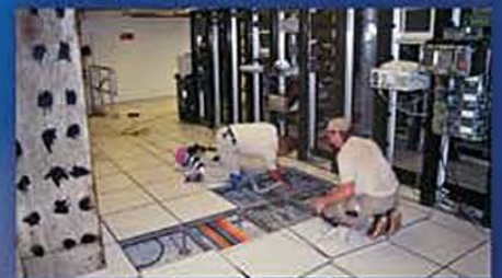
Computer Room Decontamination & Super Cleaning
