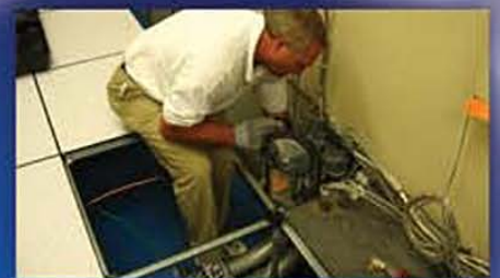
Access Panel Repair & Reconfiguration
